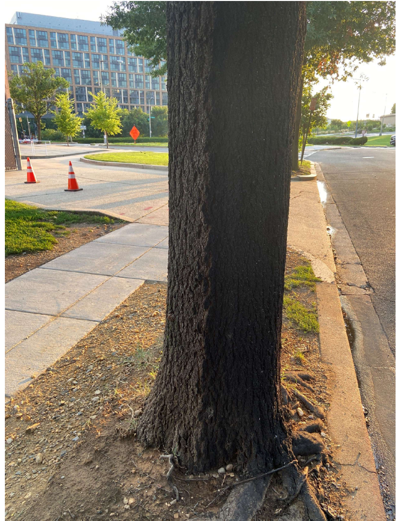
August 2022 – Fire marks still visible
